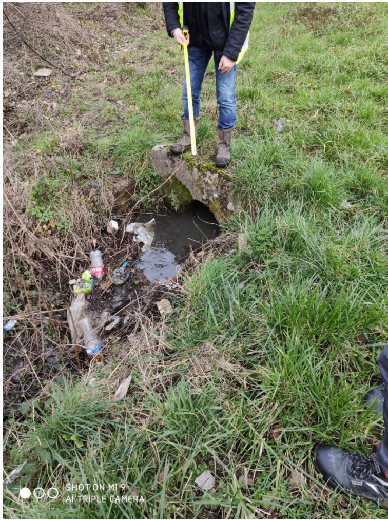
Figure 35 C:\Users\m_cha\Desktop\Heudebouville SAPN\photos\bv3\2020-02-05_15-14-55.jpg bv3 : D500 latéral RD
