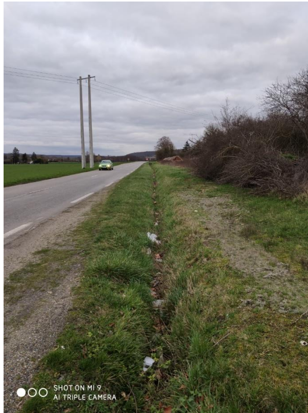
Figure 45 C:\Users\m_cha\Desktop\Heudebouville SAPN\photos\2020-02-05_17-24-50.jpg bv4 : Pinterville, fossé de la RD164
