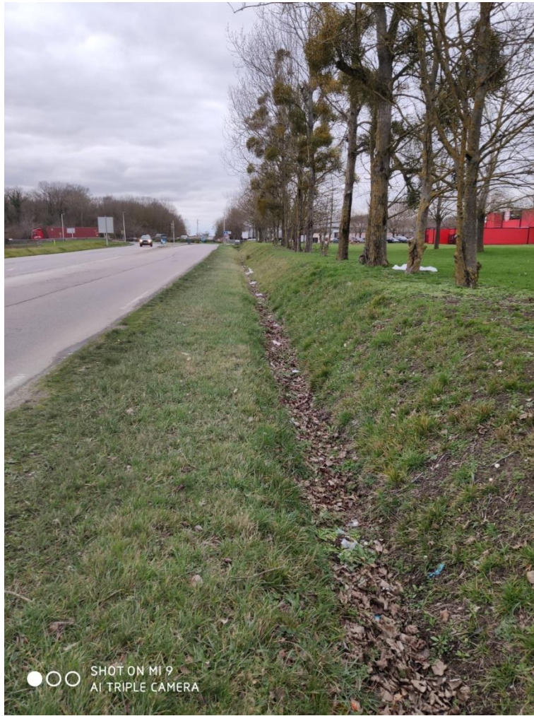
Figure 31 C:\Users\m_cha\Desktop\Heudebouville SAPN\photos\bv3\2020-02-05_16-59-42.jpg bv3 : Fossé lateral RD
